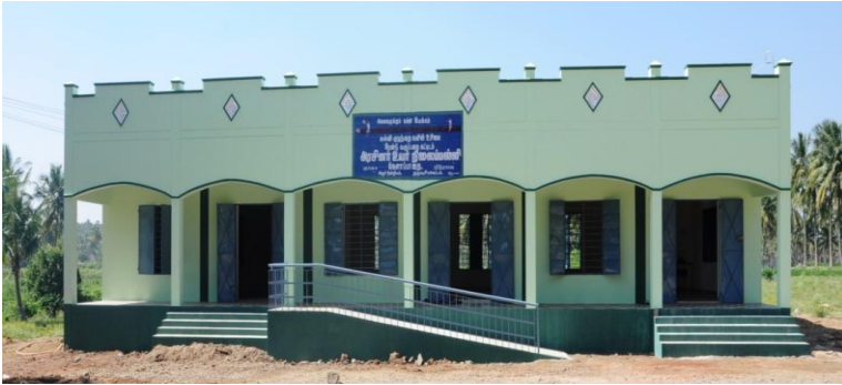
Additional Classroom Building
